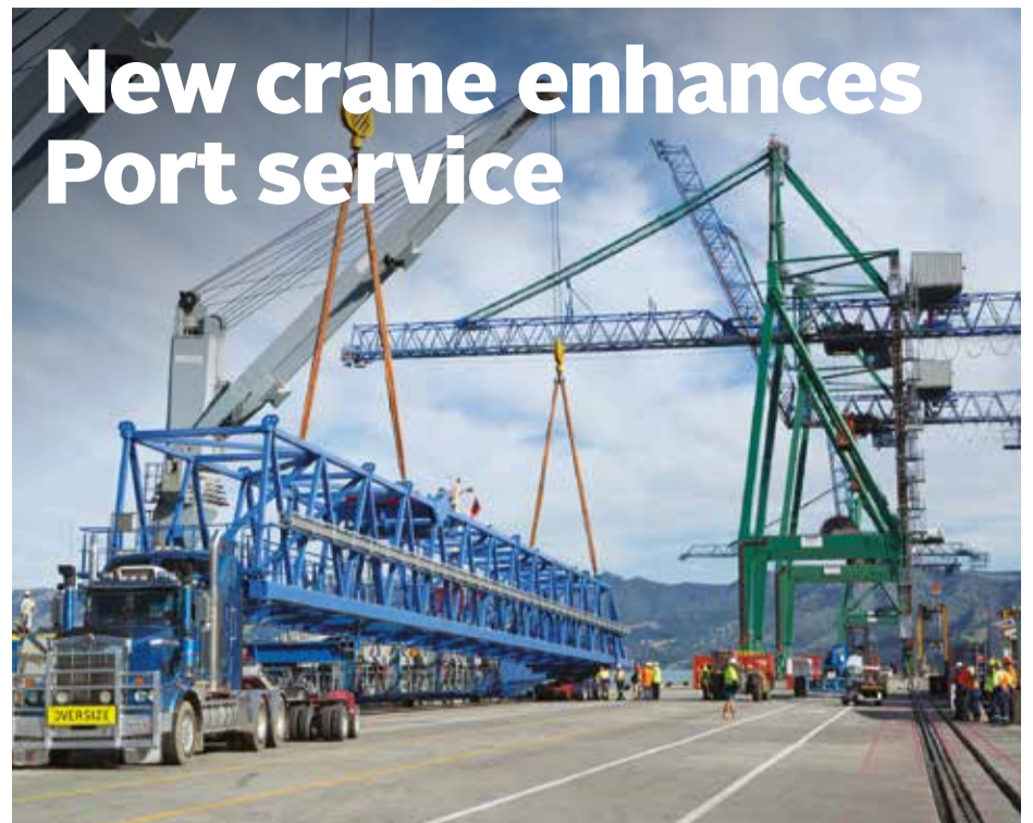
Part of the new crane arriving for assembly
