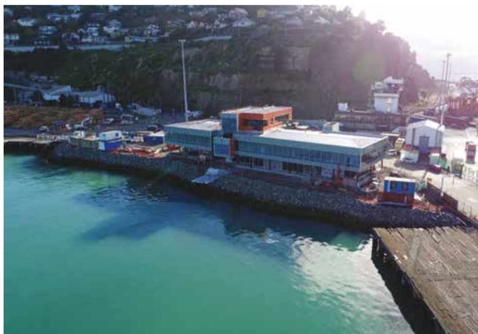
Waterfront House under construction.
