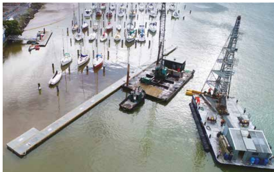
Te Ana Marina under construction.
