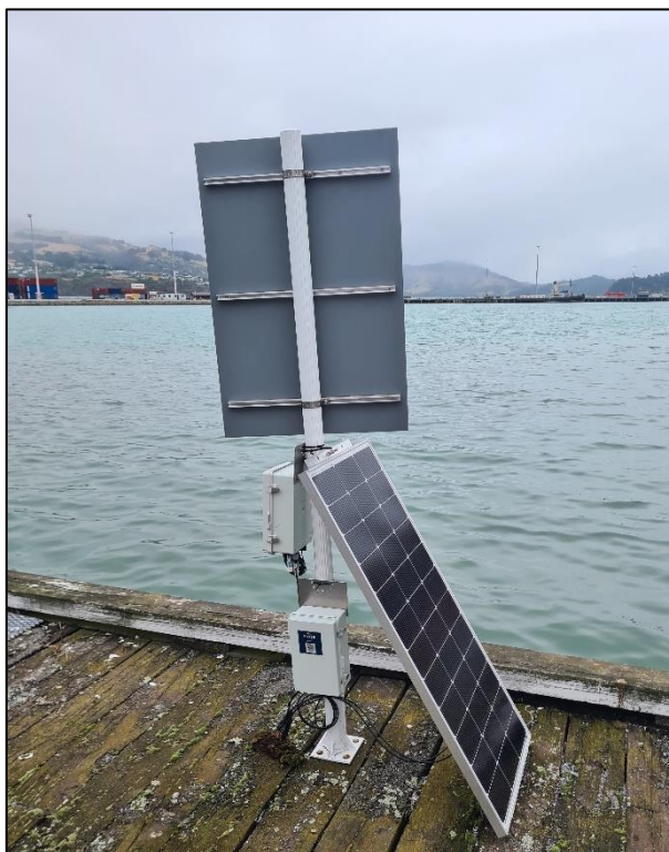
Figure 4: Installation of the PM 2.5 monitor at the end of the LPC tug boat wharf at the Port. (Image taken on 26 March 2025 looking towards the cruise berth)
